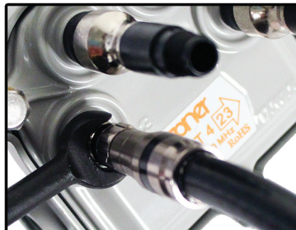
Visually inspect to ensure connector is fully compressed. Tighten to recommended torque.
